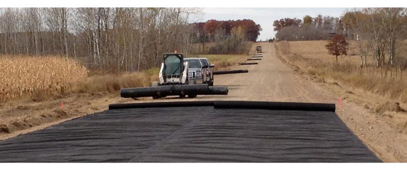
**GEOTEX®** Woven geotextiles are manufactured with high tensile strength and low elongation to provide dimensional stability and deliver superior load distribution, reducing rutting and extending the life of paved and unpaved roadways. This family of woven products offers proven performance, is compliant with AASHTO/NTPEP standards, and is available in a variety of styles to fit your specific project needs and specifications.
