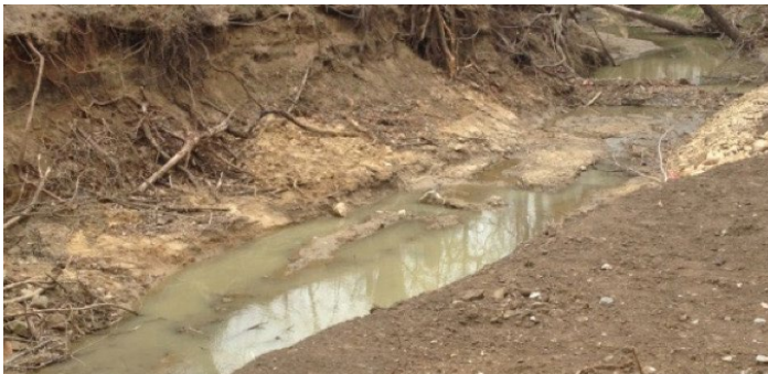
PROBLEM Heavy erosion and slope failure from frequent flooding
