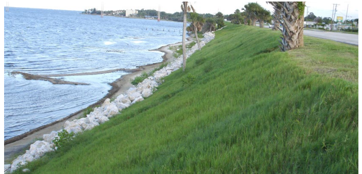
SOLUTION PYRAMAT® 75 was used to protect and maintain aesthetics
