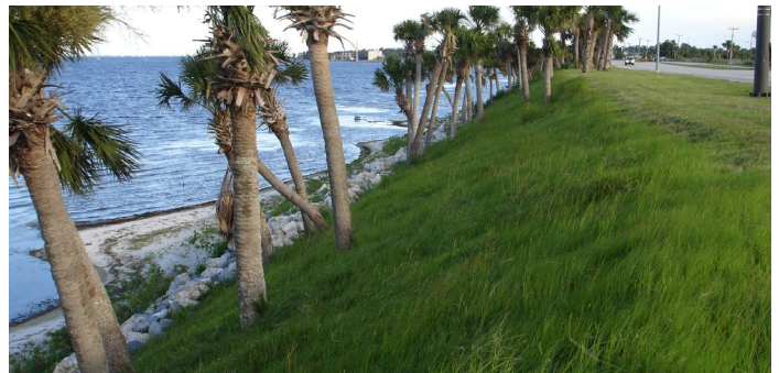
PERFORMANCE Vegetation establishment on stabilized slope
