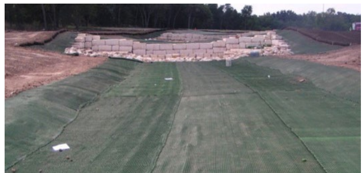
SOLUTION PYRAMAT® 75 HPTRM used to line vegetated channels over
