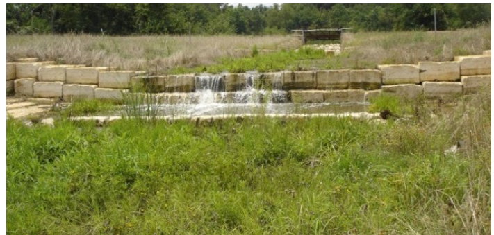
PERFORMANCE Fully vegetated, aesthetic stormwater conveyances
