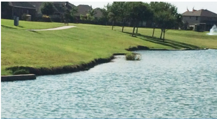
PROBLEM Pond bank erosion and sloughing due to wave action
