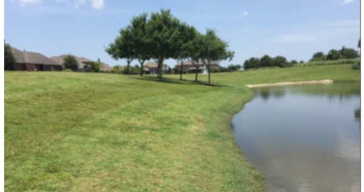
PERFORMANCE Permanently stabilized, aesthetically pleasing pond banks
