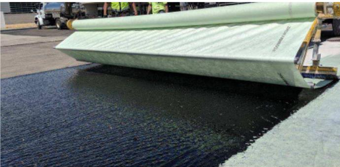
**INSTALLATION** Enviro was installed directly over a milled surface with no need of a leveling course
