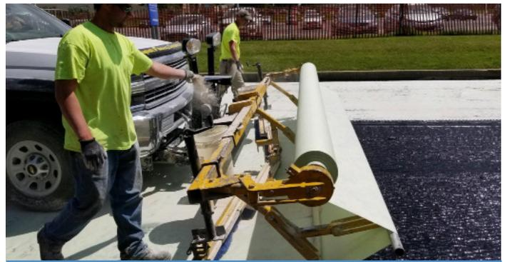
**SOLUTION** PETROMAT Enviro was selected as a paving interlayer because it can easily be recycled
