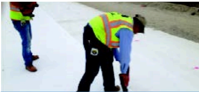
INSTALLATION REFLECTEX® was installed 6" off each side of the roadway
