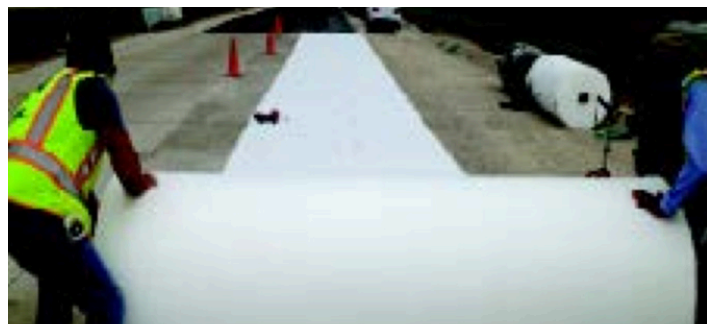
SOLUTION REFLECTEX® concrete interlayer fabric
